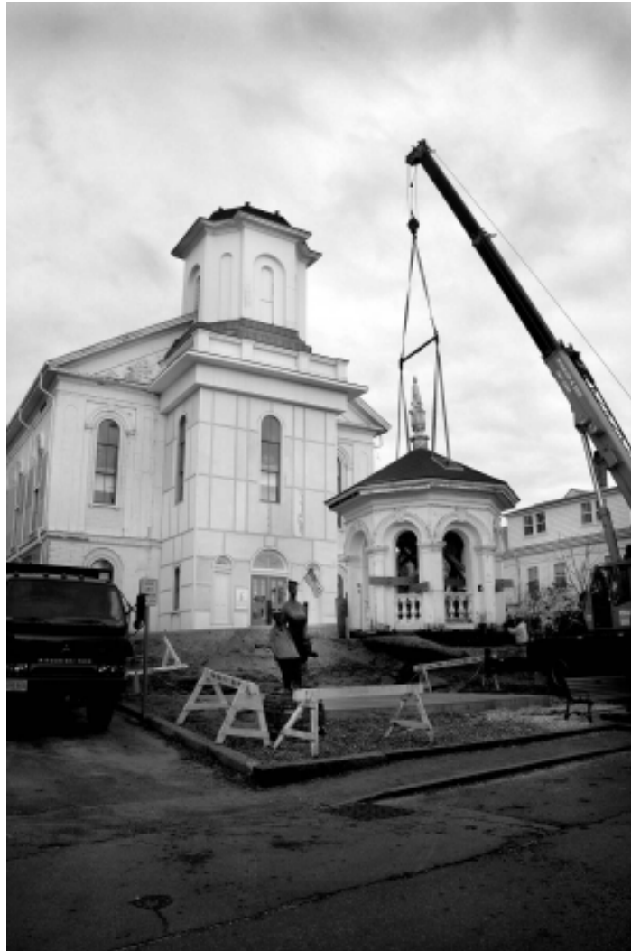
Crane moves Library belfry to temporary resting place while the structure awaits renovation and placement atop the building once funding goals are achieved.
